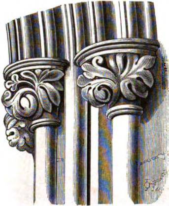
Capitals of Arch, North Aisle.
