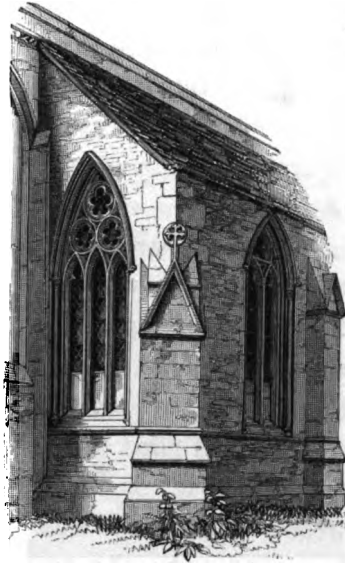
East End of North Aisle.
